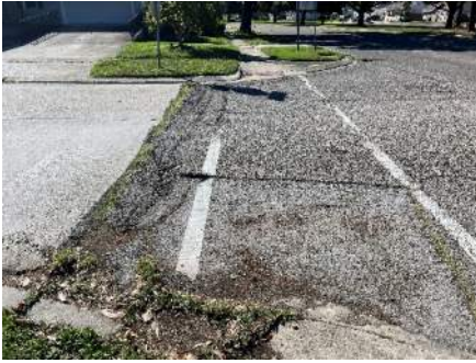
Figure 3: Turnout Deterioration
