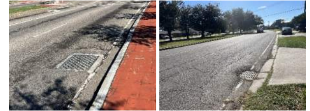
Figure 2: Drop Inlets in Road
