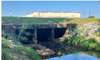
Triple Barrel Box Culvert under Downing Pines Rd.
