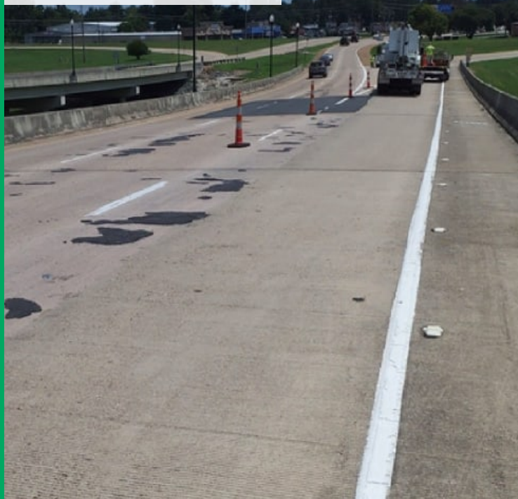
LA 3032, Bridge Resurfacing
