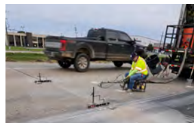
US 90 construction operations: slab jacking (left) and asphalt overlay (right).
