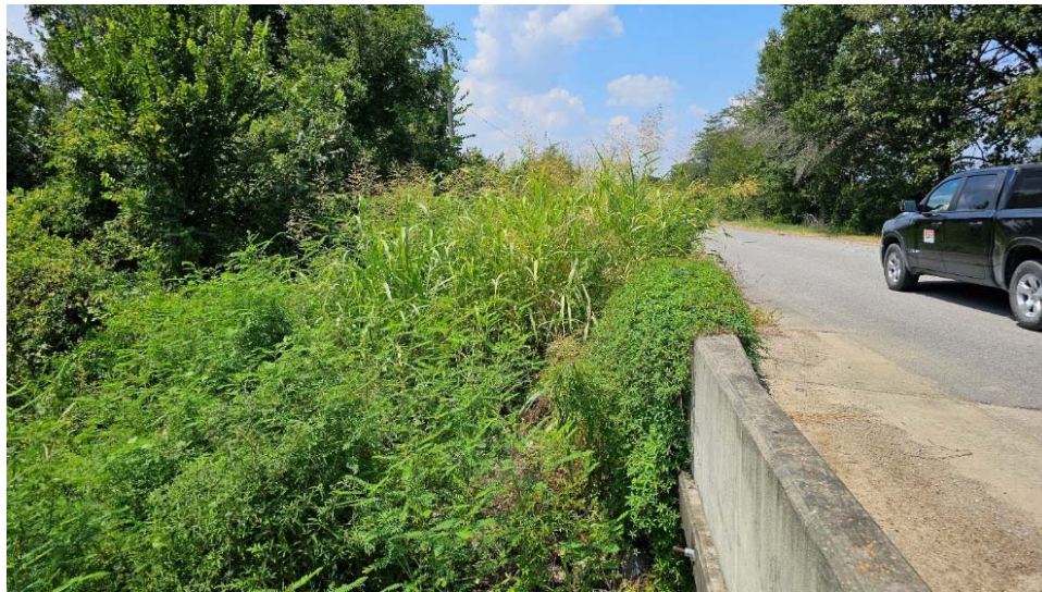
Figure 3-15: Example of In-accessible structure
