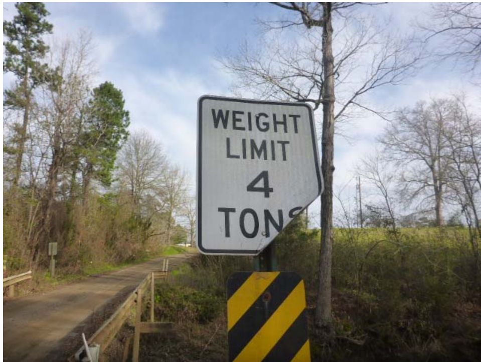
Figure 3-11: Damaged and incorrect weight limit sign
