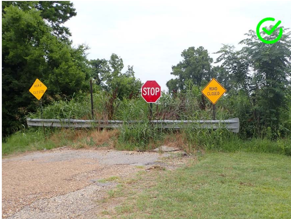
Figure 3-5: Correct closure using guardrail. NOTE: Proper signage should be used
