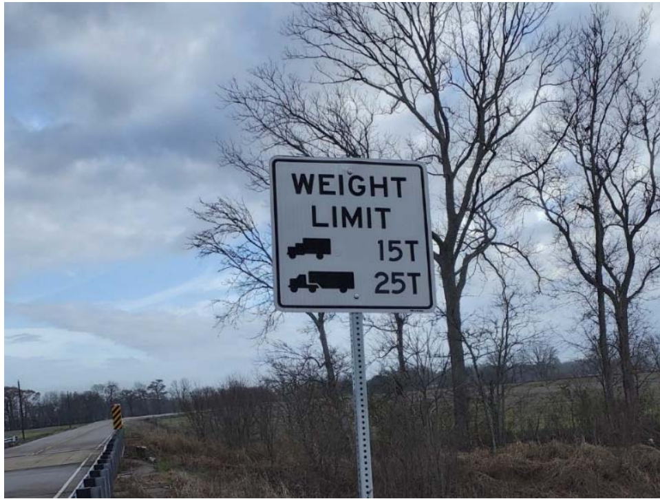
Figure 3-10: Correct weight limit sign
