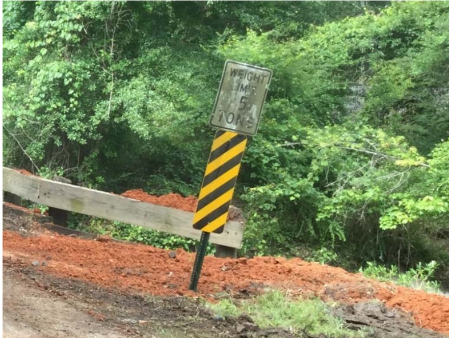
Figure 3-12: Illegible weight limit sign
