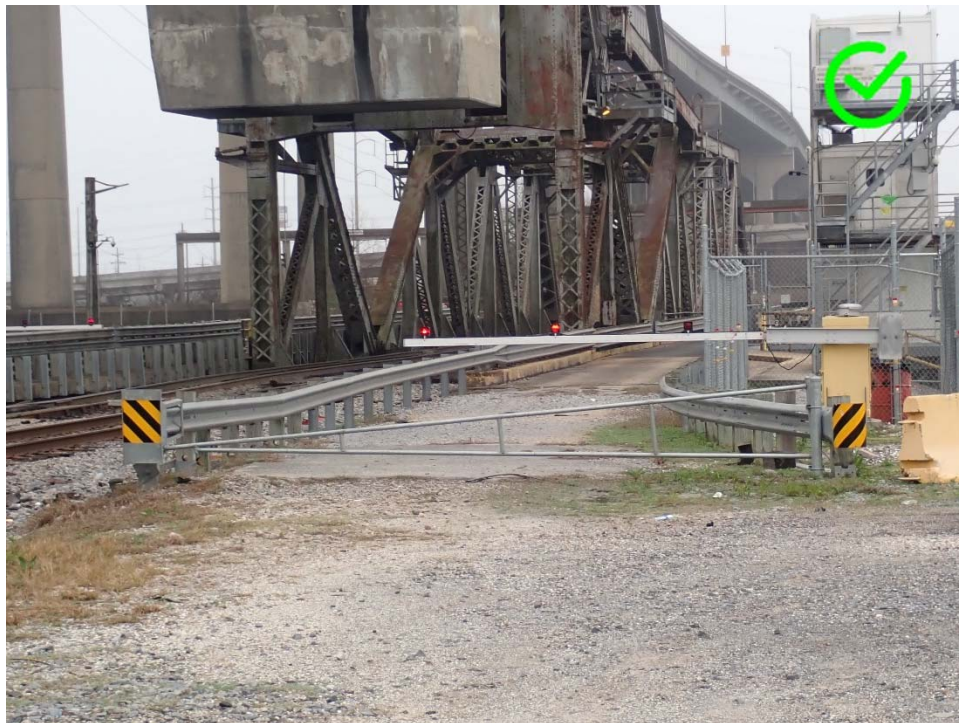
Figure 3-4: Correct closure with a locked gate
