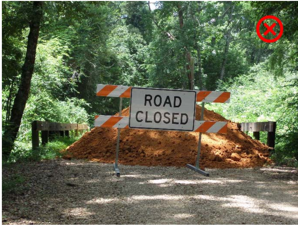
Figure 3-7: Incorrect closure using dirt pile
