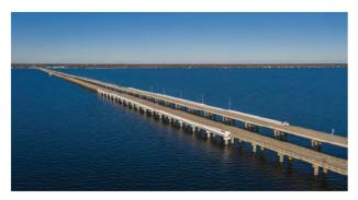
Louisiana's Lake Pontchartrain Causeway, the longest continuous bridge over water in the world, is in need of shoulders to increase safety on the bridge. Volkert was selected to design these essential and long-awaited shoulder additions. The bridge shoulders, comprising 12 bays that will provide a safe space for disabled vehicles to pull over out of traffic. They will also increase safety for motorists and emergency personnel in the event
