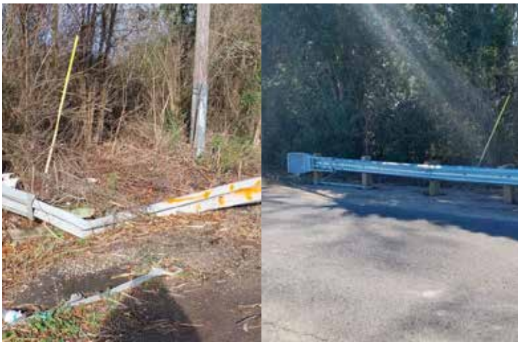
Guardrail repair before and after
