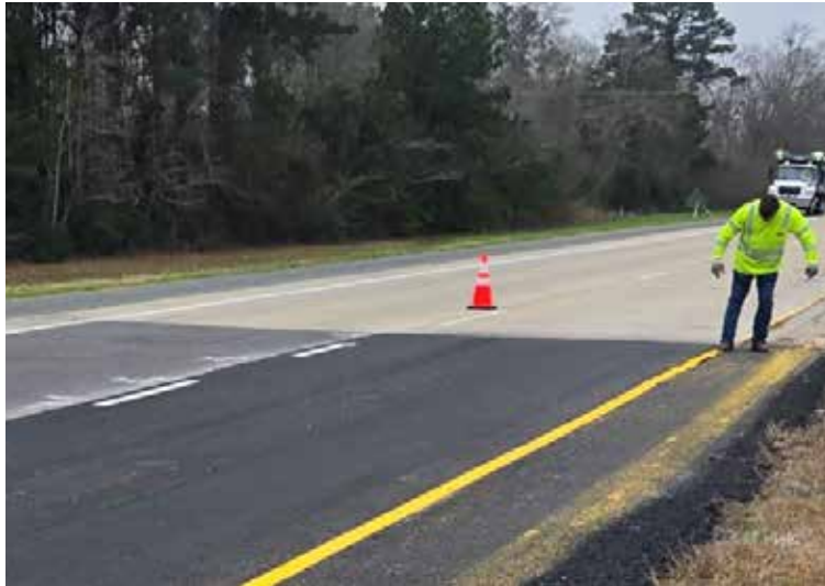
Asphalt leveling on U.S. 171 in Beauregard Parish
