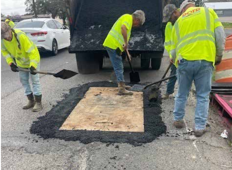
Crews installing a temporary steel plate in Acadia Parish
