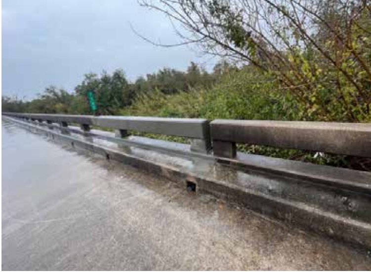
Repaired bridge rail on I-10 in St. Charles Parish
