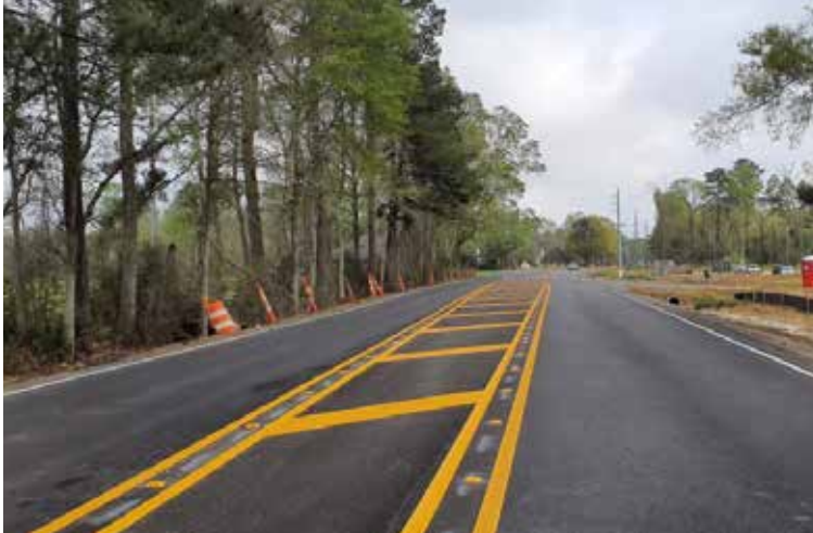
New striping in Livingston Parish
