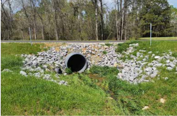
New pipe on LA 42 in Ascension Parish
