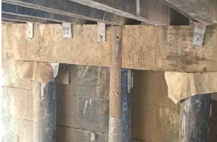
New girders installed on the bridge on LA 550 in Union Parish
