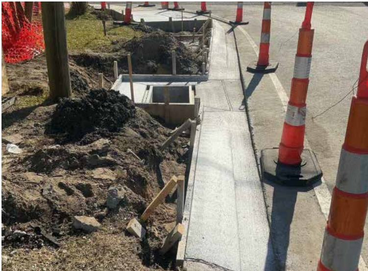
Concrete poured on LA 18 in Jefferson Parish
