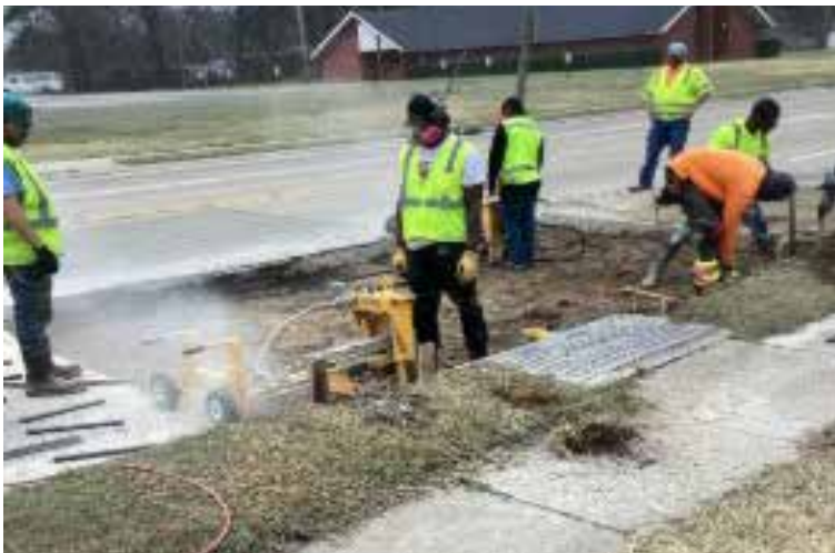
Contractors drilling tie bars for the concrete pour
