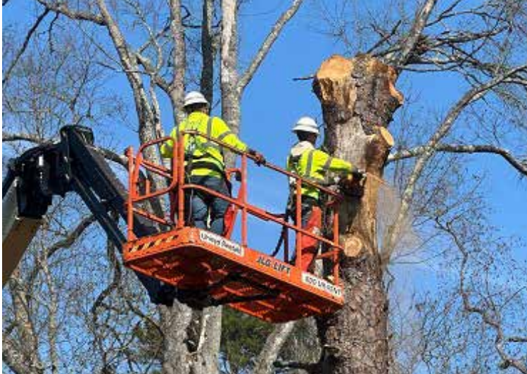
Crews cutting trees using the articulating boom manlift
