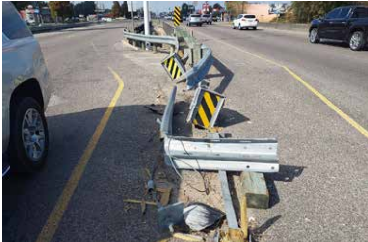
Damaged guardrail
