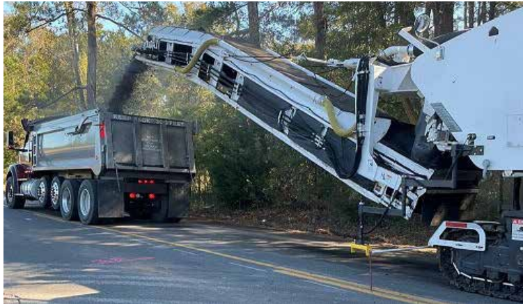
Milling on LA 120 in Sabine Parish
