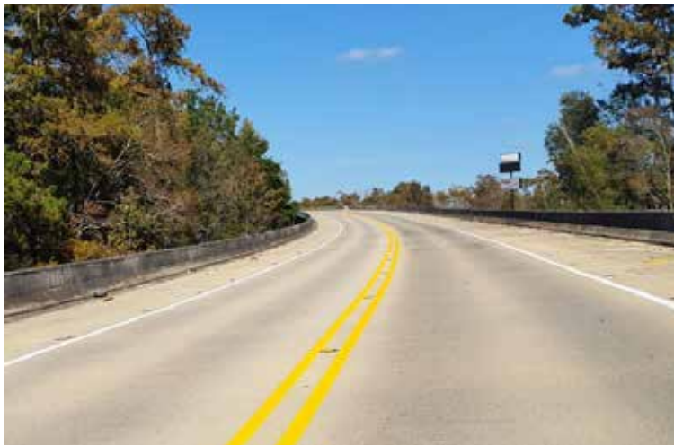
New pavement striping
