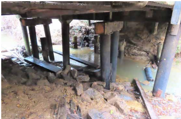
Timber piles on LA 151 in Lincoln Parish
