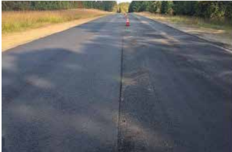
LA 9 with fresh hot mix in Claiborne Parish
