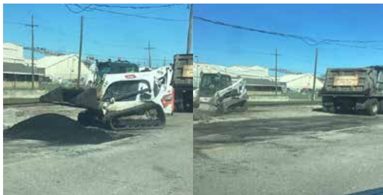
Grading patch (left) and smoothing/finishing it (right) on LA 18
