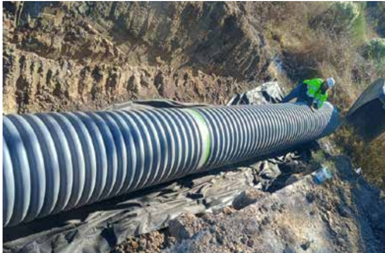
LA 134 drainage replacement in Richland Parish
