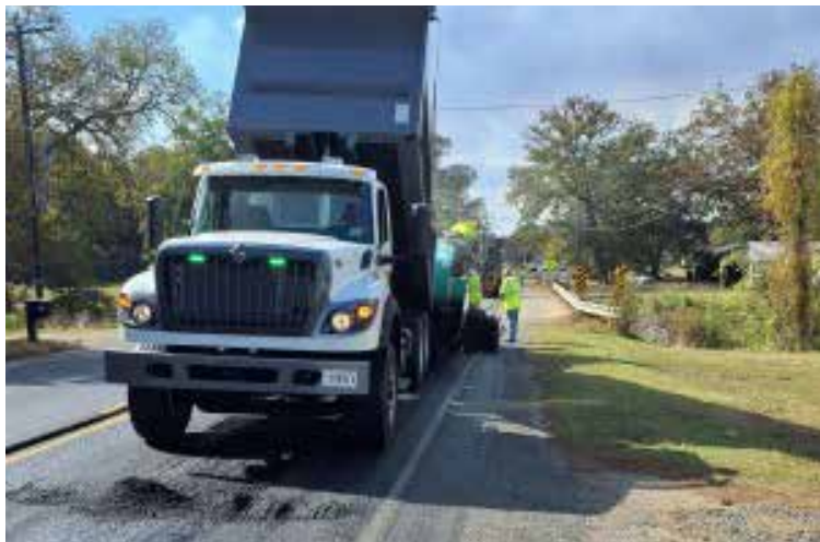
Laying hot mix on U.S. 84 in Red River Parish
