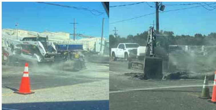
Cutting patch (left) and breaking it out (right) on LA 18
