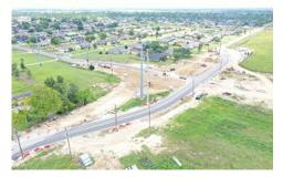
Fenstermaker worked with landscape architects to develop a sidewalk system along the corridor that immolated a park setting. The 4,700 feet of meandering sidewalk goes through an area that includes bioswales, detention areas, a tree canopy, and other green infrastructure techniques.
