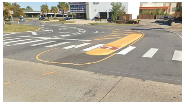
NO Ped Study: Implemented low-cost safety improvement on Read Blvd High-Visibility Crosswalk and Refuge Island
