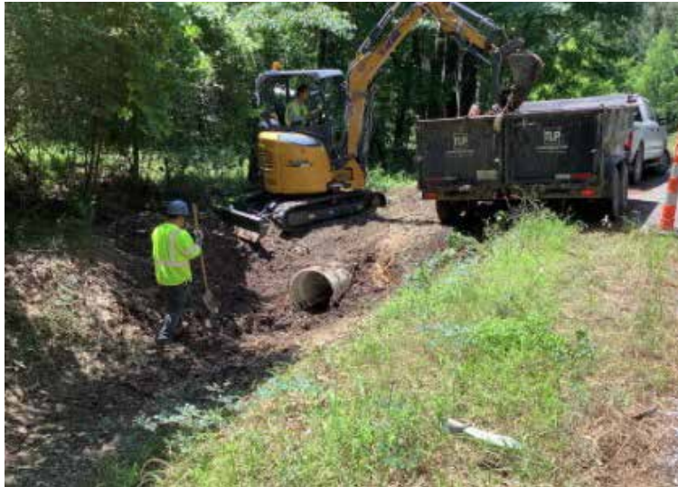
Ditch and box culvert cleaning on LA 957
