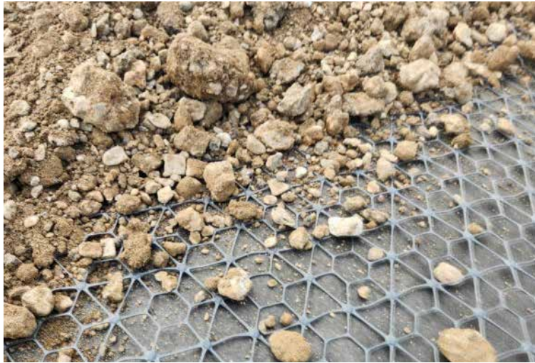
Close-up of Tensar H-Series geogrid and milled material
