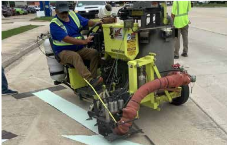
Pavement marking application on Youree Dr.
