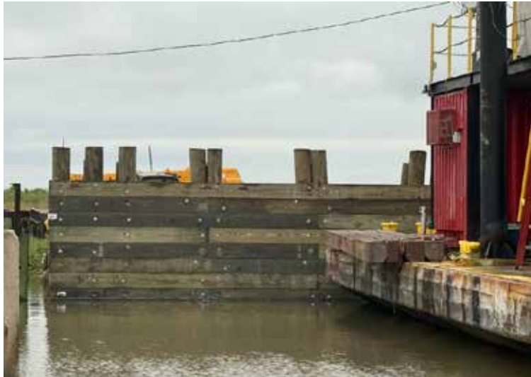
Cameron ferry's newly constructed northwest fender system
