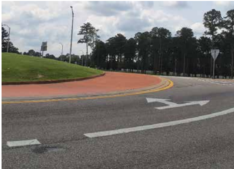
Roundabout striping
