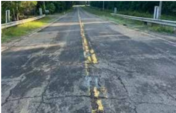
Condition of LA 507 before overlay in Red River Parish
