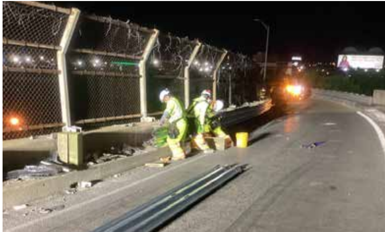
Guardrail replacement in the New Orleans area
