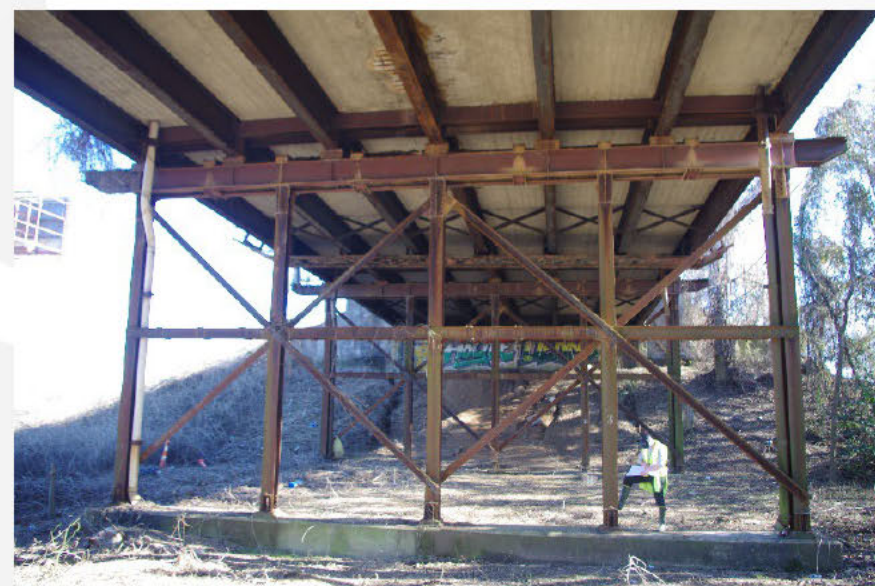
Linwood Avenue Bridge over Railroad Tracks - Typical Bent
