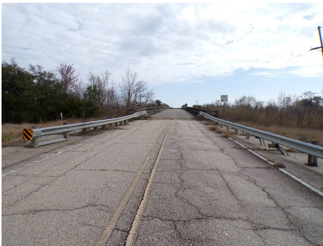
Photo 7: West Middle Pearl River Bridge
