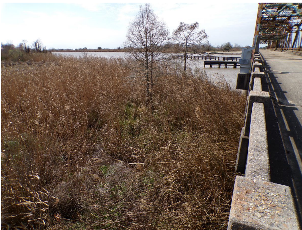
Photo 22: East Pearl River Bridge
