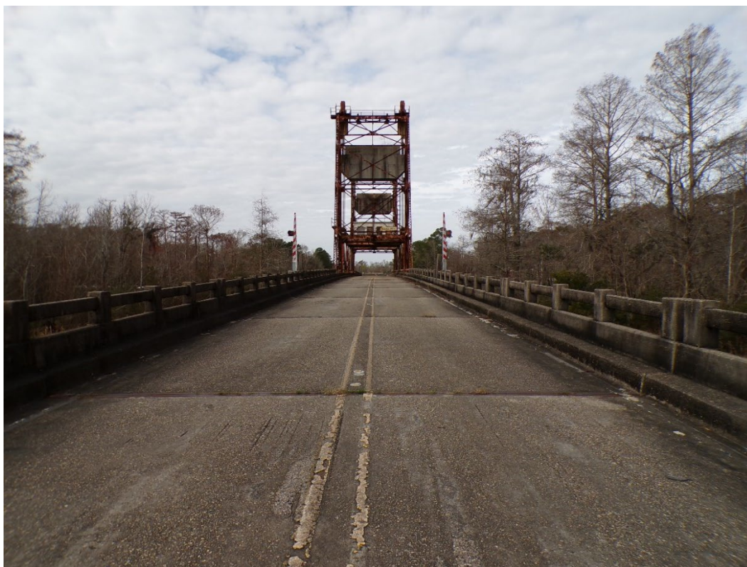
Photo 1: West Pearl River Bridge
