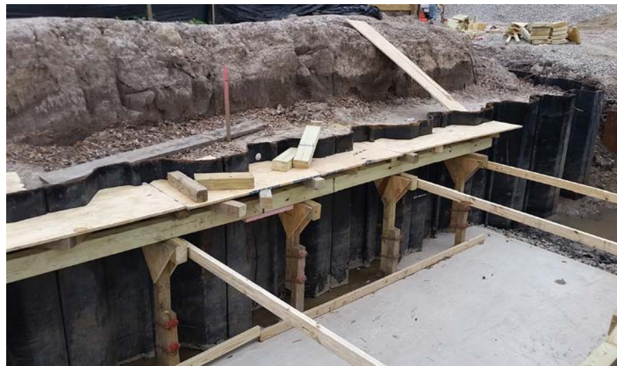
Cast-in-Place Concrete Dry Bottom
