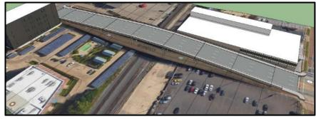
lengths ranging from 80 ft. to 90 ft. At a design speed of 30 mph, grades are 6.2% and -6.5%.
