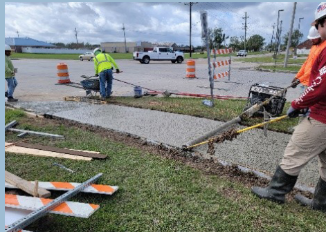
Figure 3. Our team provides consistent on-site presence throughout all phases, enabling real-time quality assurance and swift resolution of construction challenges.
