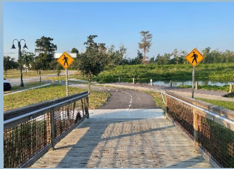
Figure 1. Thompson CE&I on a levee multi-use path project involving the levee, ped bridges, and safety features.
