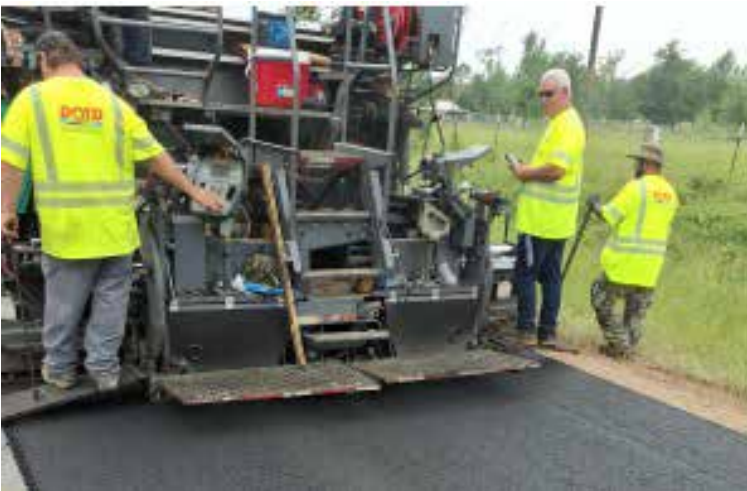
Crews working on LA 175 in DeSoto Parish
