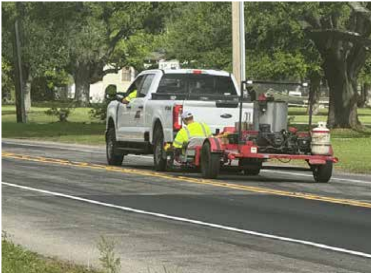
Applying reflective buttons on LA 308 in Lafourche Parish
