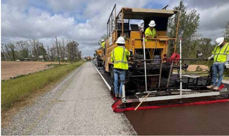
U.S. 84 microsurfacing project in Catahoula Parish
