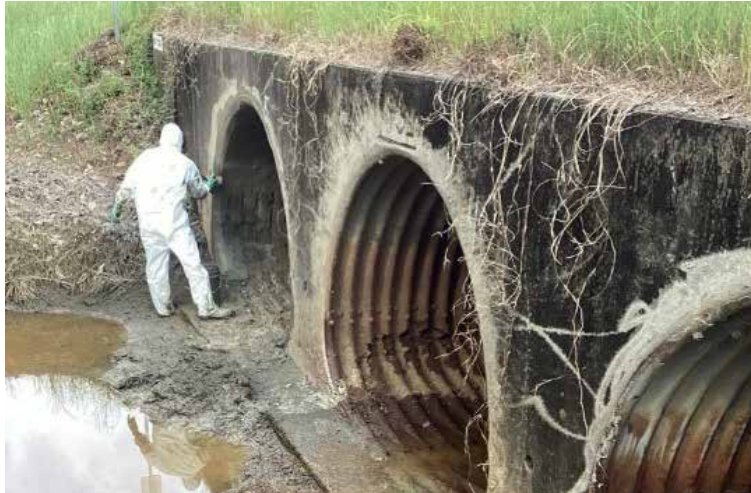
Culvert rehabilitation in Beauregard Parish
