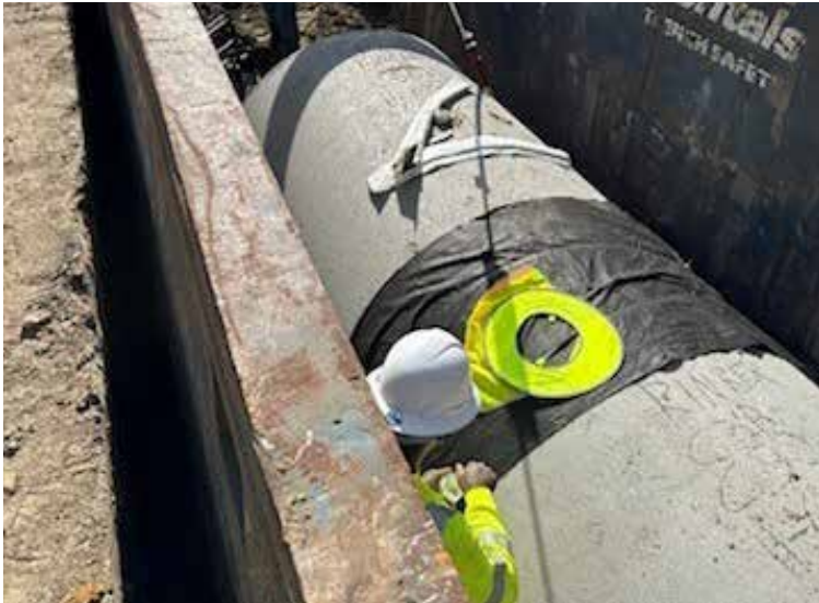
LA 13 cross-drain replacement in St. Landry Parish
