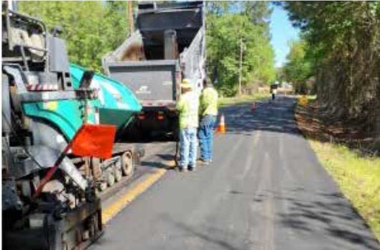
Hot mix on LA 788 in Red River Parish
