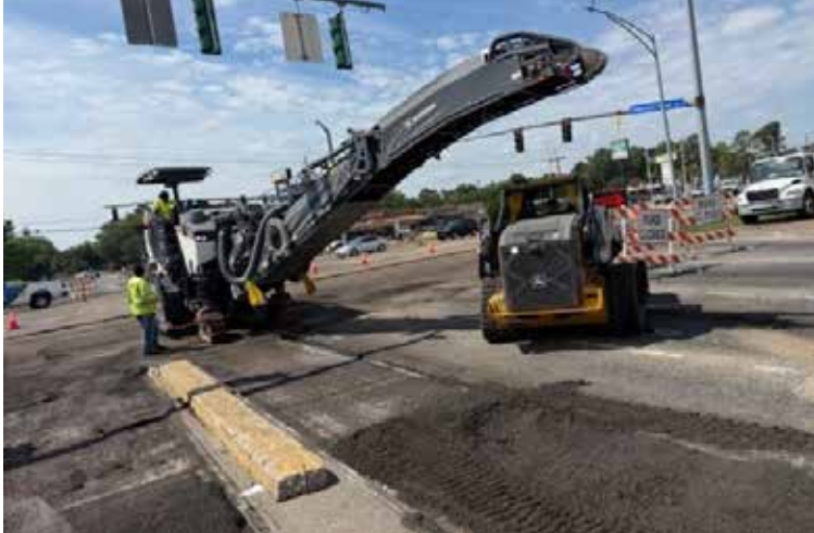
Fresh asphalt on U.S. 190 in East Baton Rouge Parish
