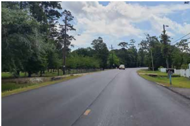
New asphalt on LA 433 in St. Tammany Parish
