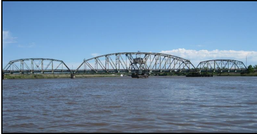
View Upstream Approach, East Pearl River Bridge
