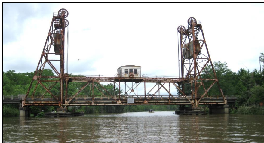
View Upstream Approach, West Pearl River Bridge
