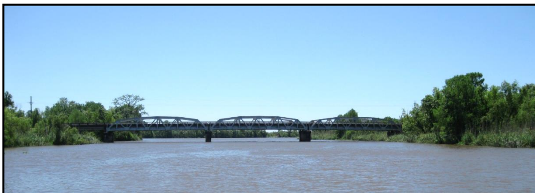
West Middle River Upstream Approach
