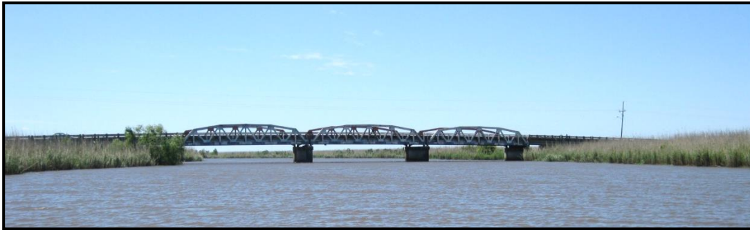
Middle Middle River Upstream Approach
