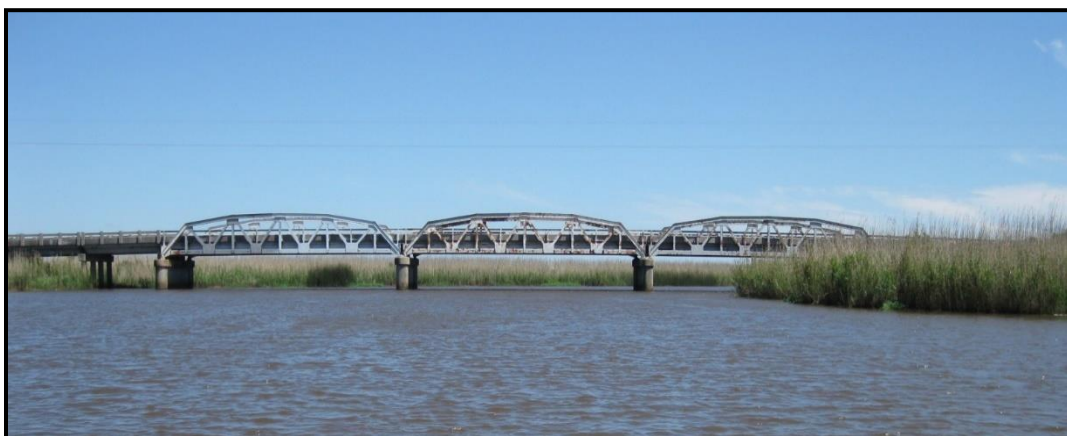
East Middle River Downstream Approach
