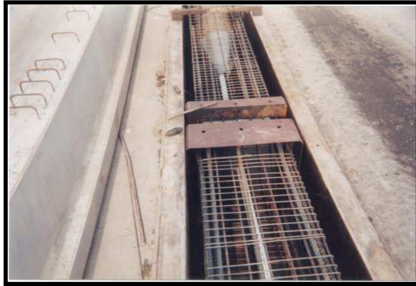
Splice Integrated with Steel Reinforcement during Fabrication
