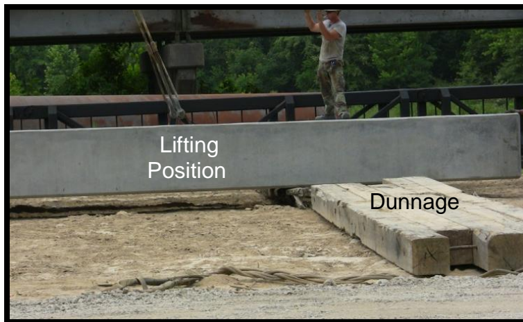
Pile Placed Incorrectly on Dunnage
