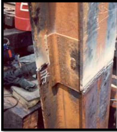
Steel H-Pile Splice
