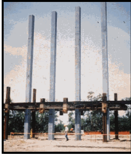
Single-Tiered Template with Piles
