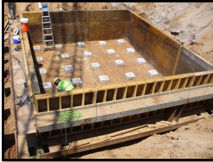
Concrete Pile Group for Footing
