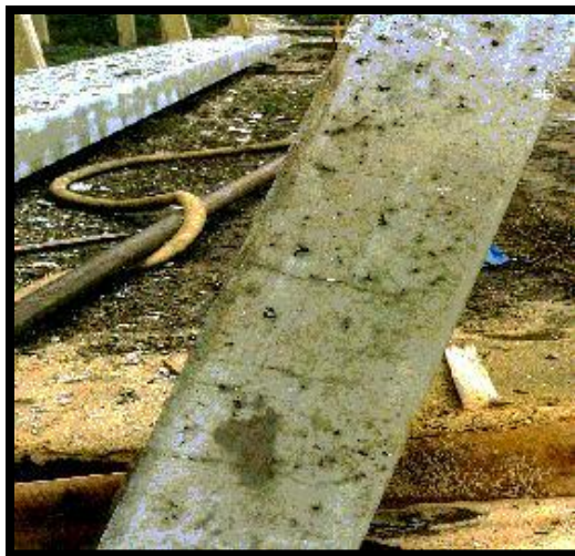
Example of micro cracks
