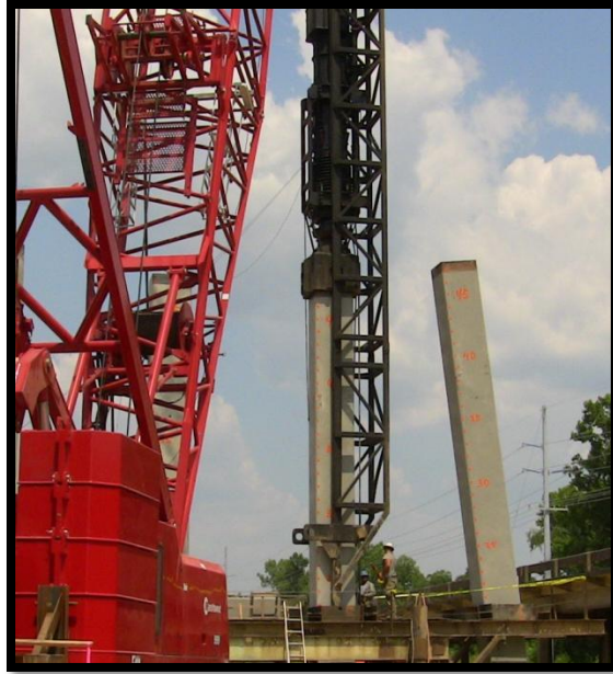
Box Lead Supporting Hammer and Pile
