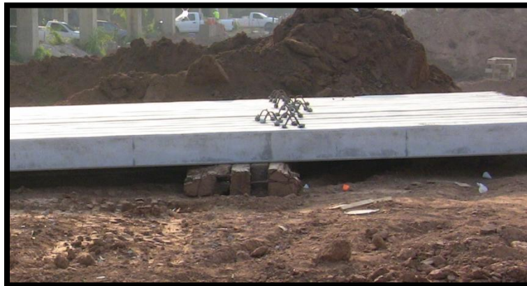
Piles Placed Properly on Dunnage
