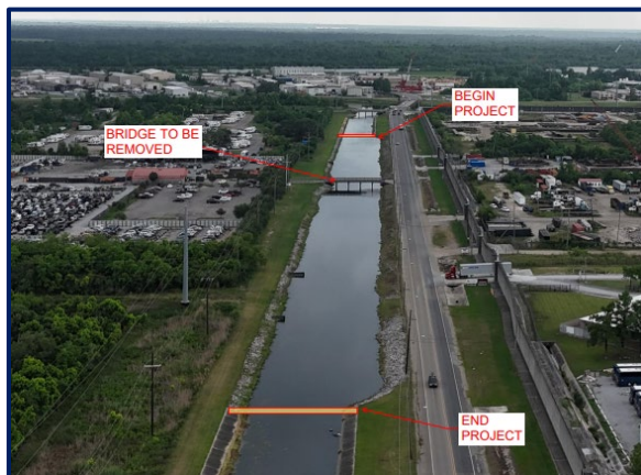
Aerial view of the project corridor along LA 3017 and Murphy Canal illustrating the constrained work area, parallel alignment of roadway and canal, and proximity to adjacent properties.
