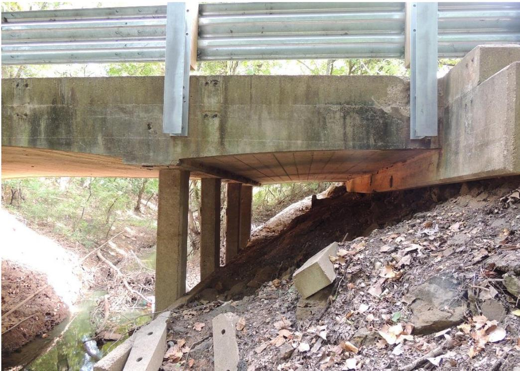
*Character-defining Feature Photo 1: The north span of the Red Bayou Bridge, with concrete pier caps integrated into the haunched concrete slab superstructure, which results in a monolithic continuous slab design.*
