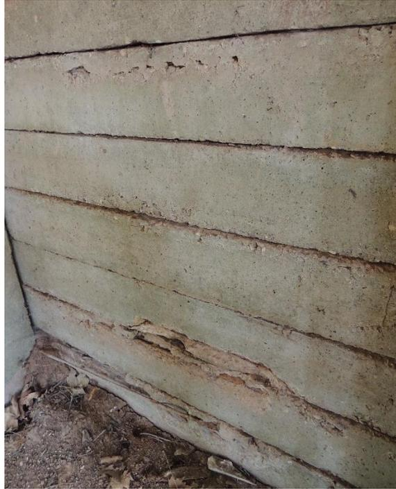
*Condition Photo 8: Concrete spalling with exposed reinforcing steel at the crib wall at bent 3.*
