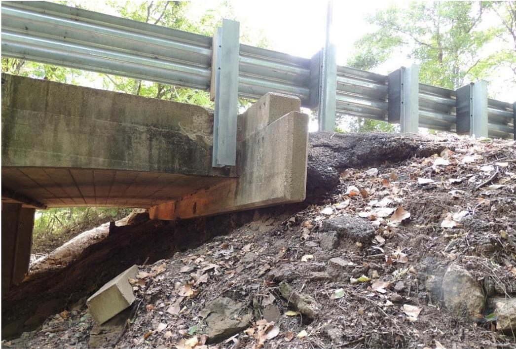
*Condition Photo 12: Bent 1, west wingwall, erosion and undermining of the approach roadway.*
