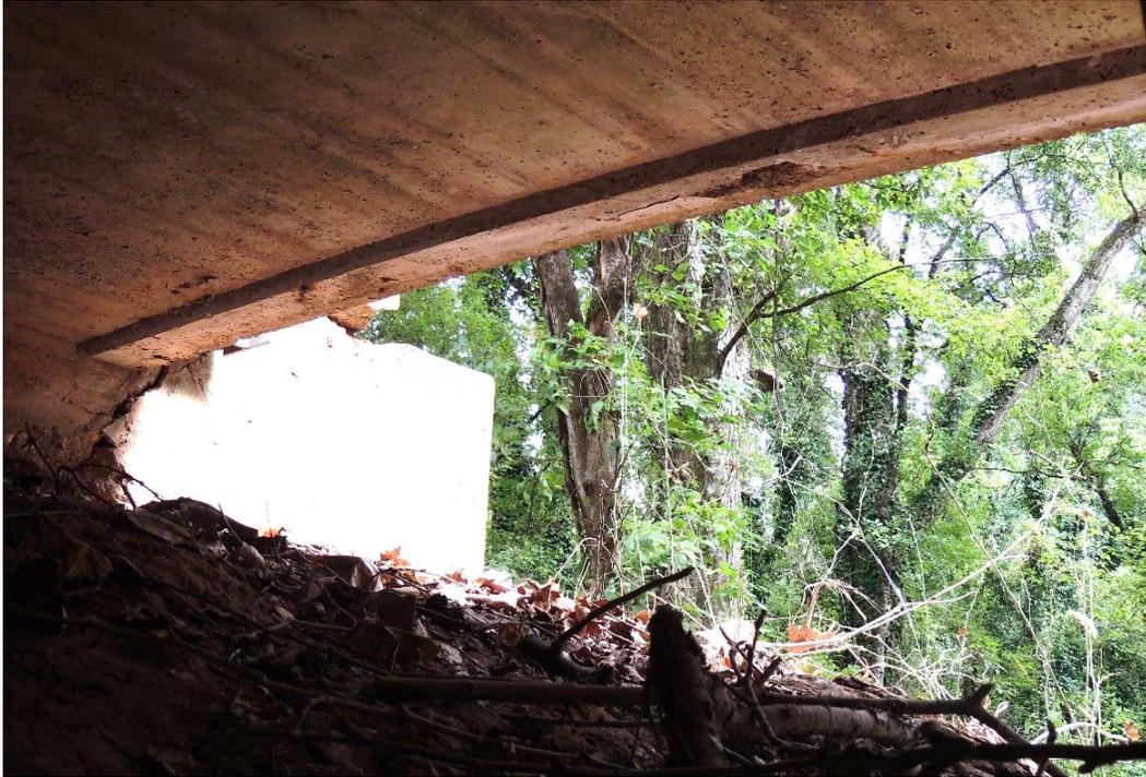
*Condition Photo 6: Concrete spall with exposed steel on the underside of the span 2 slab.*
