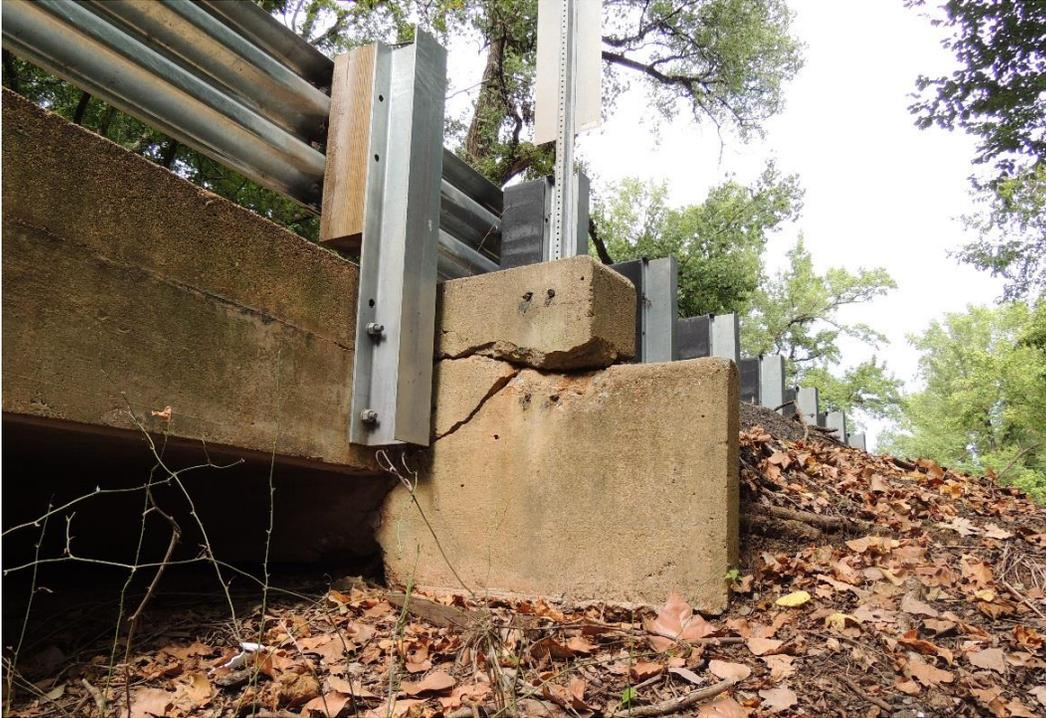
*Condition Photo 4: Bent 4, east wingwall cracked and spalled with exposed steel, looking north.*
