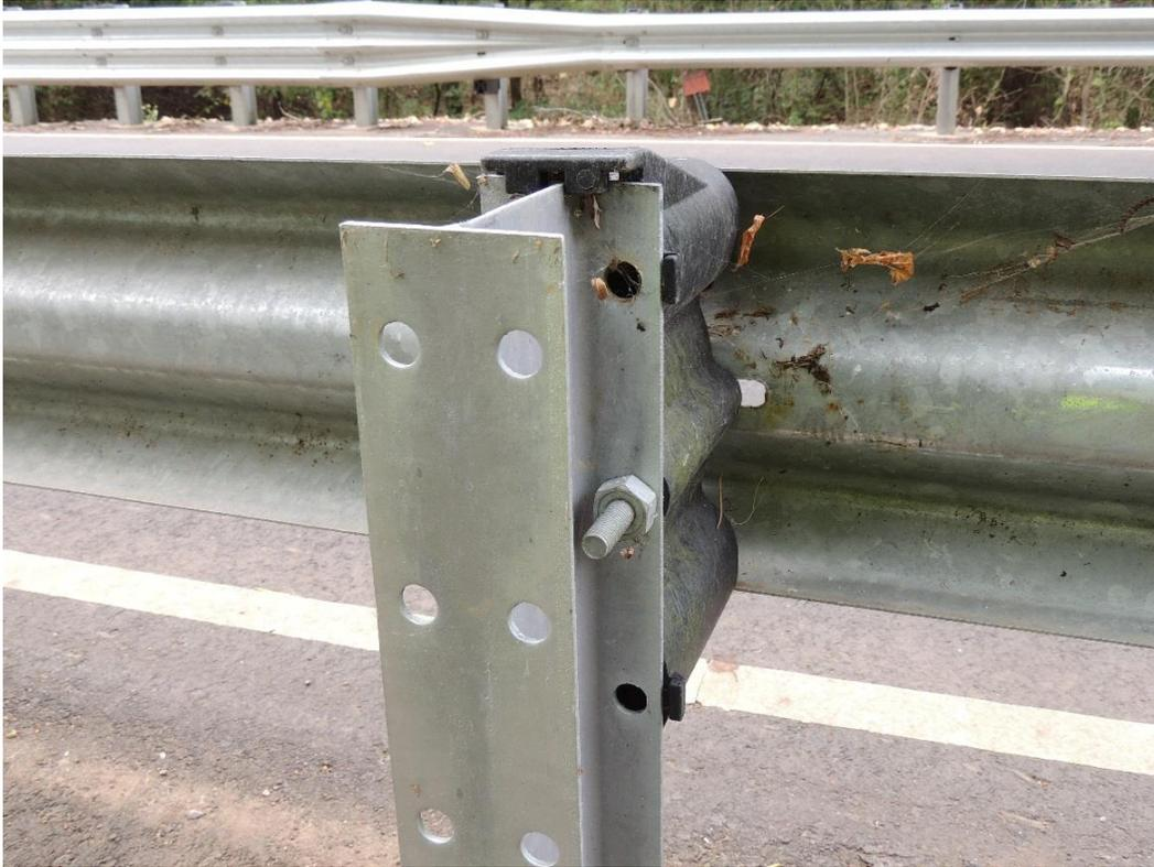
*Condition Photo 10: Rubber blocking for the guardrail connection along the roadway approach.*
