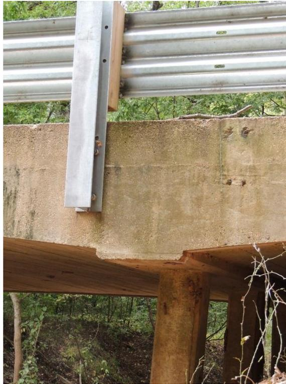
*Character-defining Feature Photo 2: Close-up view of integrated pier cap poured monolithically with the concrete slab.*
