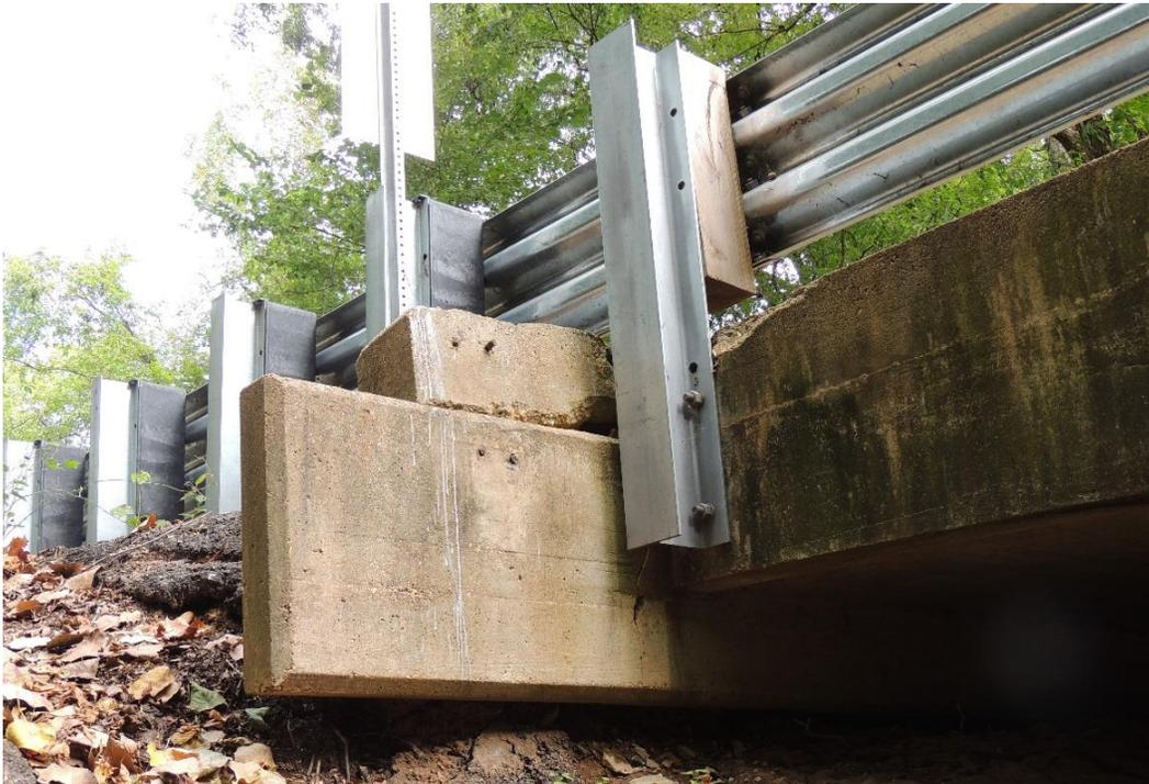
*Condition Photo 11: Bent 4, west wingwall, erosion and undermining of the approach roadway.*
