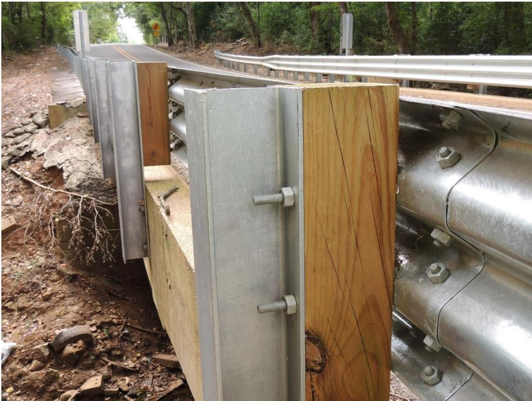
*Condition Photo 9: Timber blocking for the guardrail connection along the bridge.*
