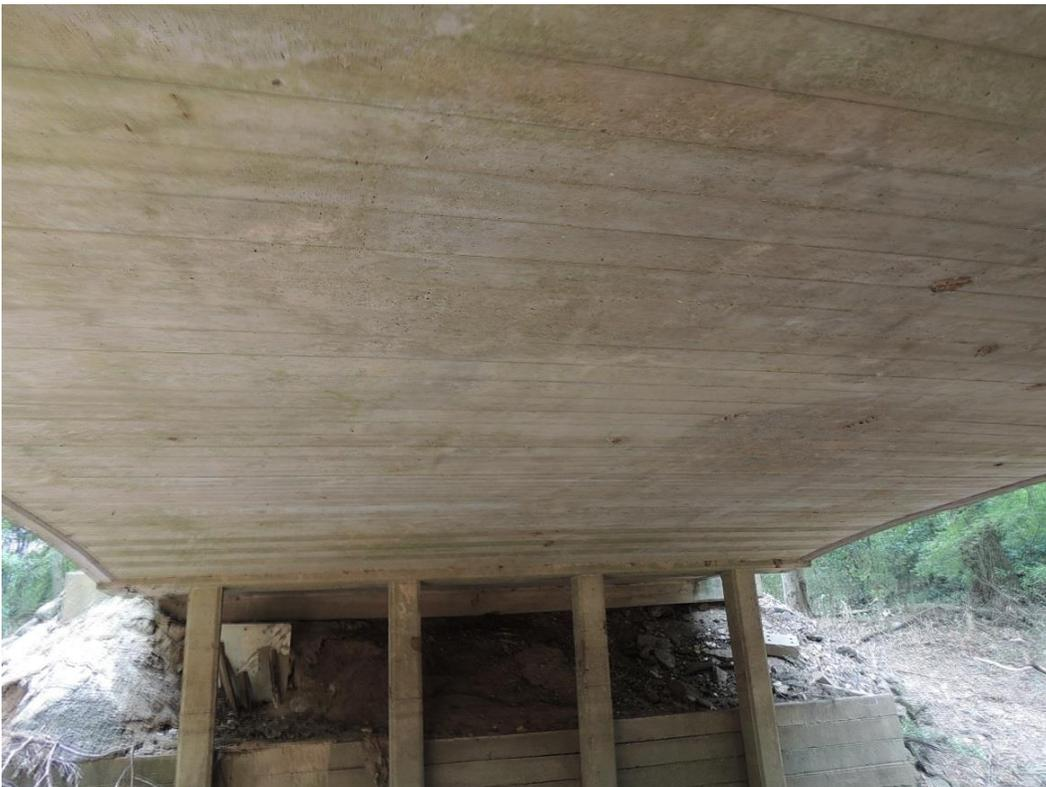
*Condition Photo 5: Concrete honeycombing on the underside of the span 2 slab, typical condition.*
