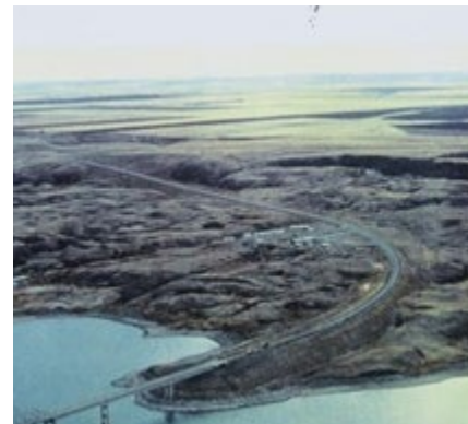
Figure 1 (left) – Aerial View of Forest City Landslide
