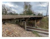
The two bridges at Minden, LA serve as part of the I-20 interchange at US 371. The bridges were built at different times around 1930 and both bridges are three span, steel girder bridges. One bridge is normal skew to the roadway
