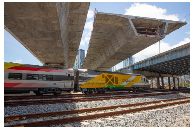
Brightline Rail Crossing under I-395
