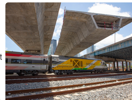
Figure 3. Segmental Cantilever over Railroad
