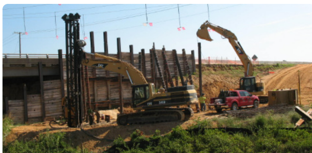
Short Length Pile Splicing near Railroad
