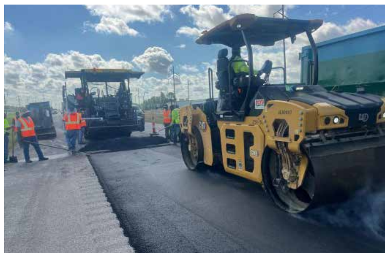
Patching on U.S. 61 in East Baton Rouge Parish
