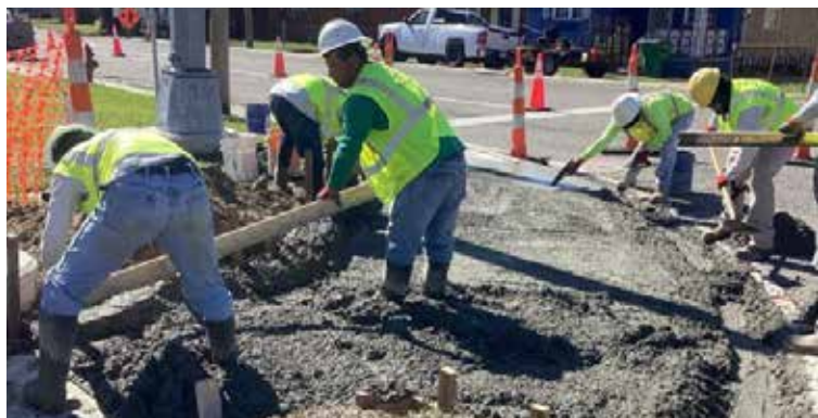
Pedestrian curb ramp installation in Westwego
