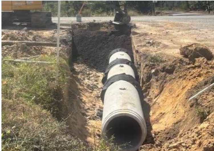
Cross drain extension on LA 10 in Allen Parish
