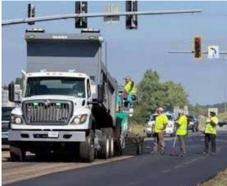
Capital outlay project in Acadia Parish
