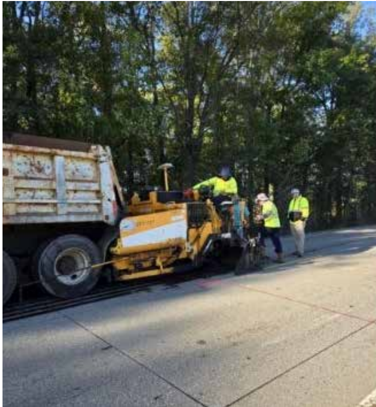
Asphalt crews working on U.S. 80 in Madison Parish
