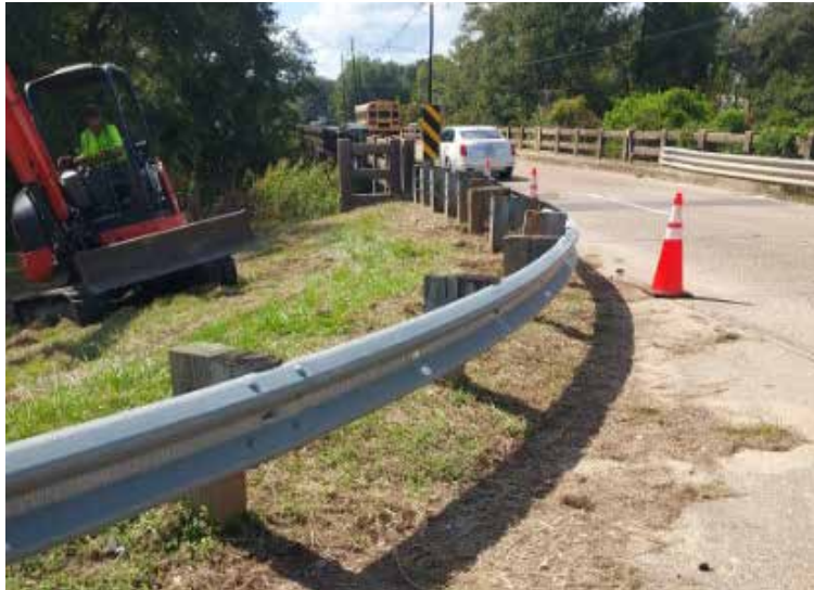
Newly repaired guardrail
