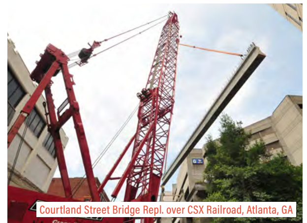
Courtland Street Bridge Repl. over CSX Railroad, Atlanta, GA
