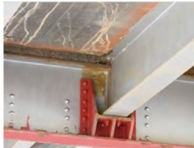
Figure 2: Existing steel girder saddle.
