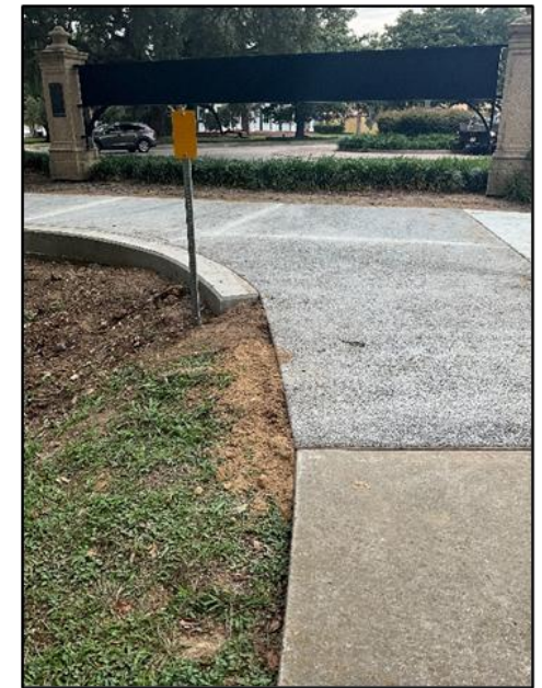
Completed Pervious Pavement H.009290 – LSU
