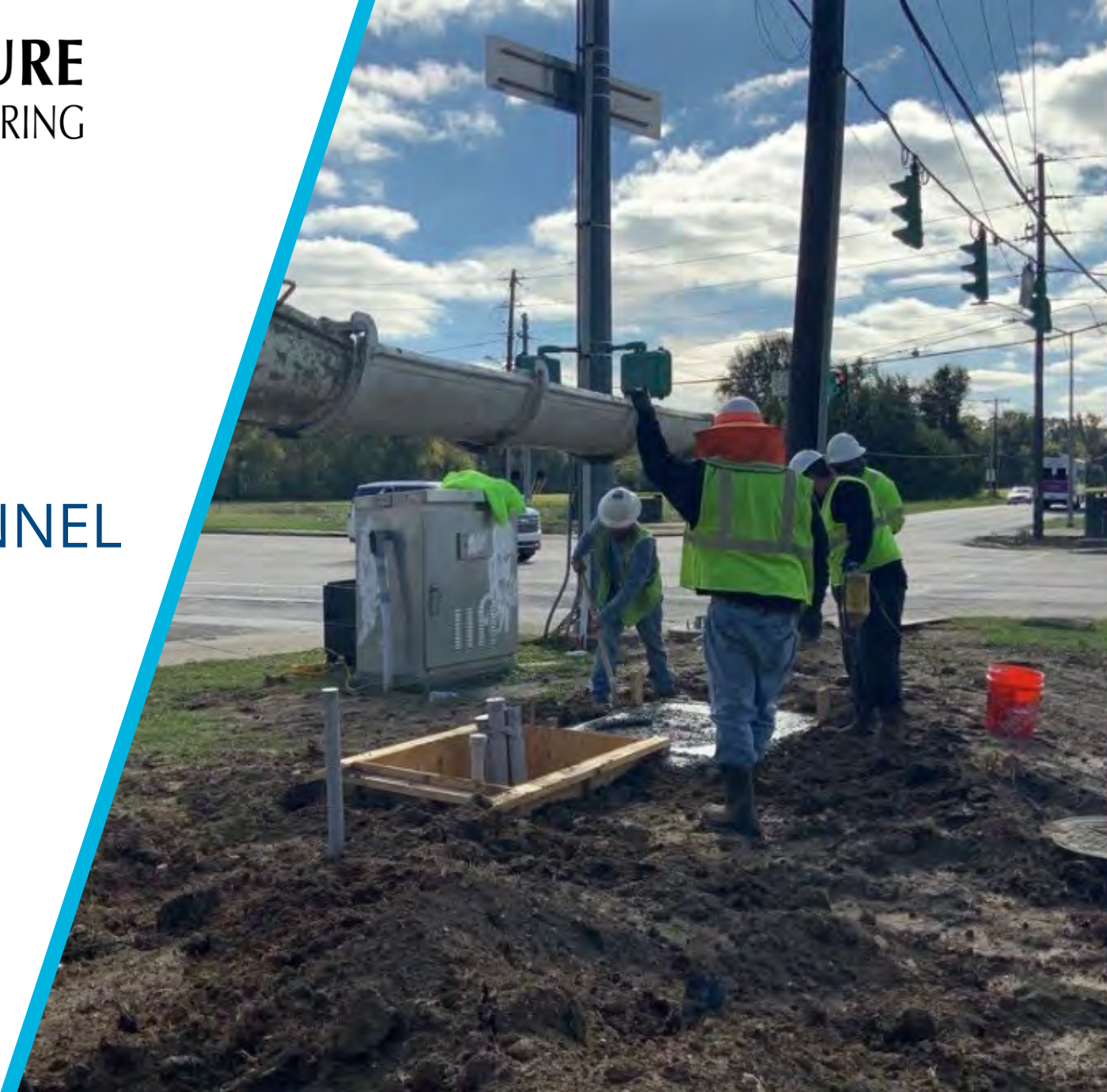
Signal Installation and Field Inspection
