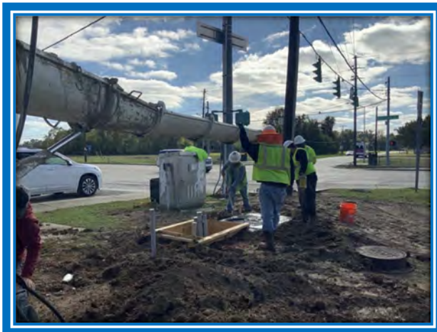
Signal Foundation Installation : Lafayette, LA
