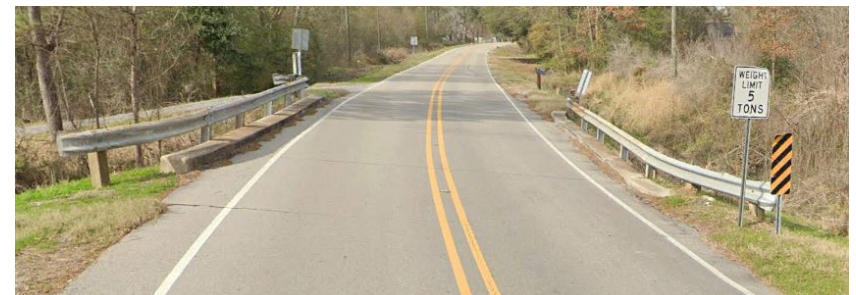
EXISTING EAST FLANCHER RD. OVER DRAINAGE CANAL
