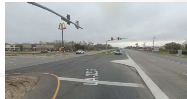
Figure: Implemented Continuous Green-T Intersection Concept at LA 3235 and LA 3162
