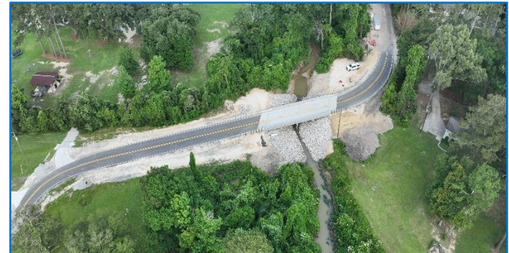
Wildwood Drive Bridge over Beaver Creek Post Construction Photo
