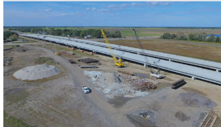
US 90, LA 318 Interchange DB (Geoengineers)
