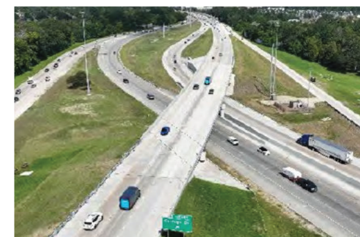
Photo of realigned I-12 WB through lanes to more closely follow the I-12 EB existing alignment along with new I-10 flyover bridge
