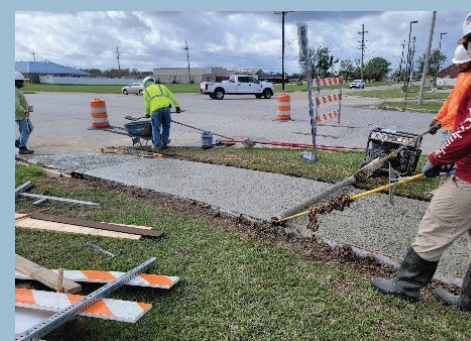
Figure 3. Our team provides consistent on-site presence throughout all phases, enabling real-time quality assurance and swift resolution of construction challenges.
