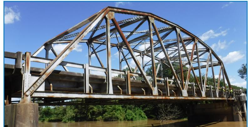
Once the load rating was accepted by MDOT, the inspection reports were updated to account for any adjustments in the fracture critical member schematic.
