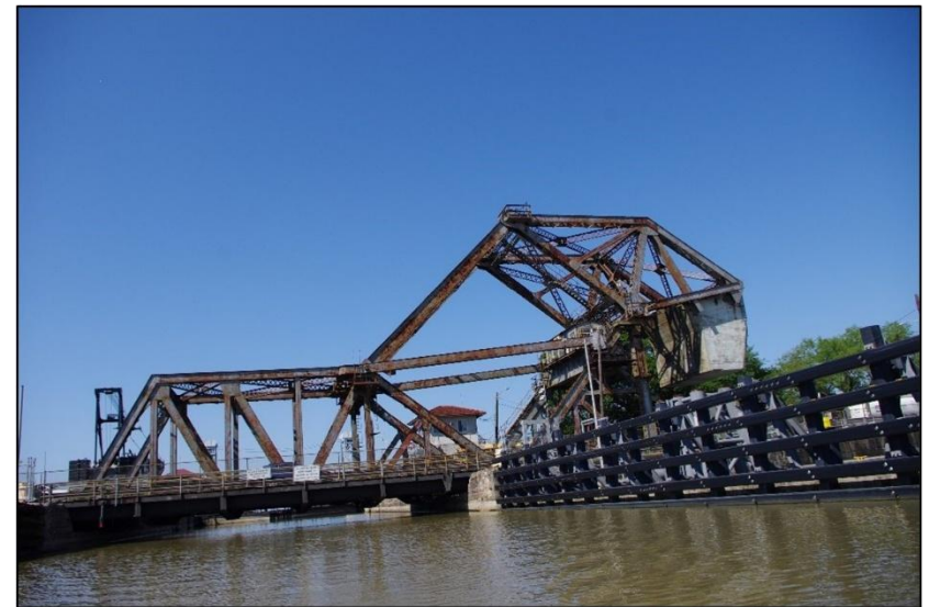
St. Claude Bridge owned by Port of New Orleans Inspected and Load Rated
