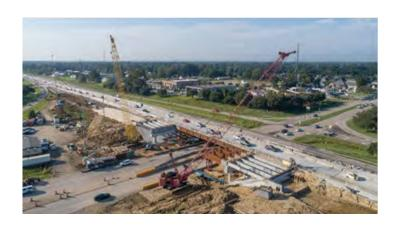
In order to maintain high volume traffic on I-10 while reconstructing the bridge, the new bridge had to be constructed in 3 separate phases.
