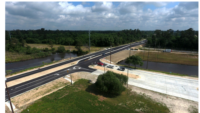
Completed four-lane roadway section with raised median
