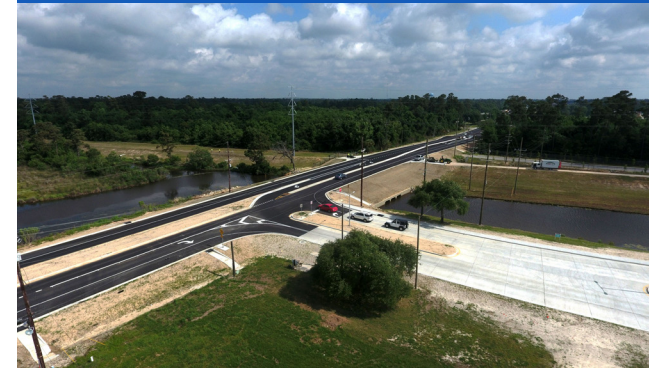
Completed project view of US 11 improvements
