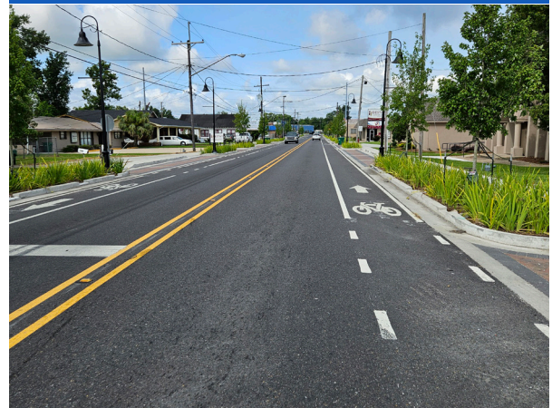
Completed road improvement project with bike lanes and new sidewalks
