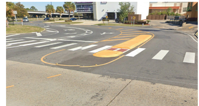
NO Ped Study: Implemented low-cost safety improvement on Read Blvd High-Visibility Crosswalk and Refuge Island
