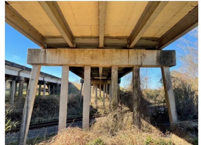
US 190 UPRR Overpass – WB Pile Bents and Girders
