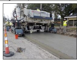
Street reconstruction project. Replacement of all underground utilities (water, sewer, and drainage) and construction of new wider PCCP pavement. Project included detailed sequences to monitor access to residents over this 20-block-long project.
