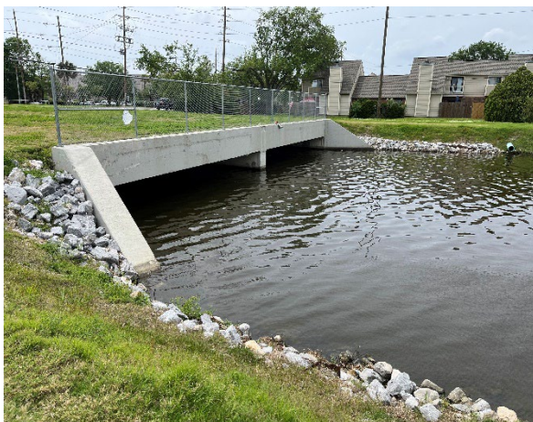
Figure 3: W. Esplanade Bridges at Duncan Canal
