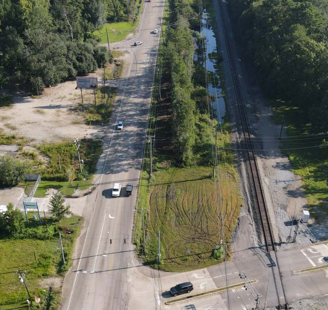
North Boulevard at US 11 and NSRR
