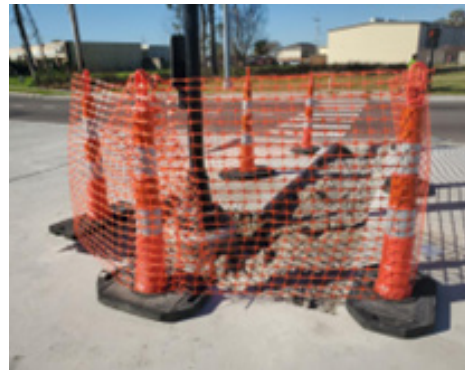
Ped Pole/Ramp installation H.011670 Kenner
