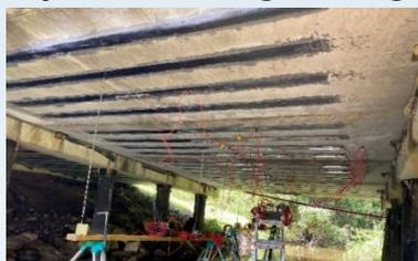
Precast slab bridge rehabilitated with standard detail provided by WSP during the SCDOT load rating contract.
