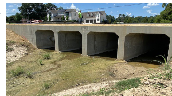
New box culverts in Manchac Acres, Ascension Parish.
