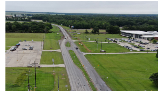
Drone photo of intersection of LA 3211 and Yokley Road and surrounding area
