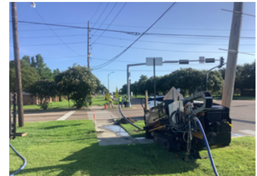
Boring conduit for conductors for pedestrian signals at intersection of Vintage Drive and Loyola Drive
