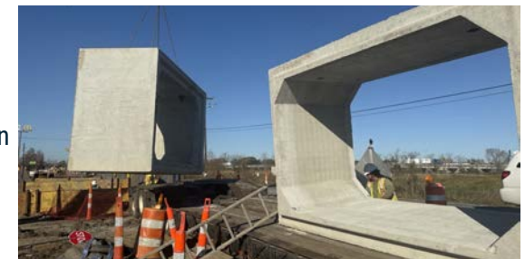
Installation of new drainage structures for LA 352.
