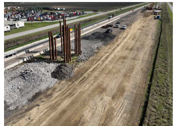
Test pile and approach work.
