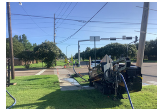
Sidewalk construction on Vintage Drive
