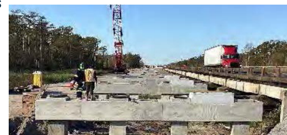
I-10 Widening & Bridge Replacements east of Coone Gully.
