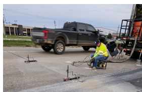
US 90 construction operations: slab jacking (left) and asphalt
