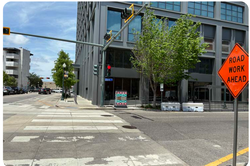
New traffic control boxes will protect new wiring for the new pedestrian signals. Coordination with CVU and the City will be needed to protect the decorated City assets.
