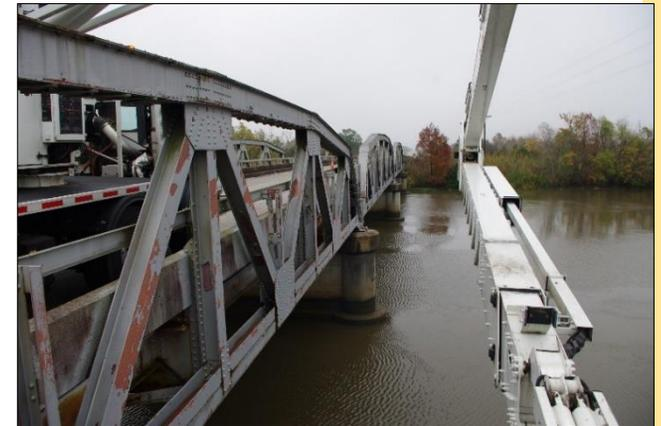
*Complex Truss Bridge Being Inspected for Load Rating Analysis*
