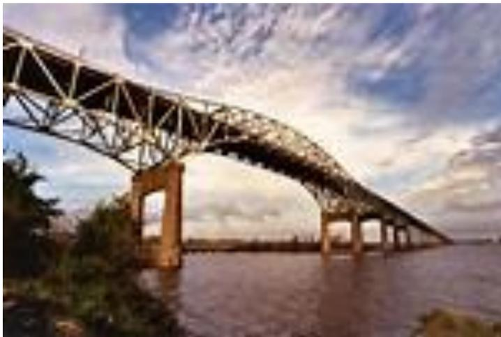
The I-10 Calcasieu River Bridge carries I-10 over local roads, railroads, and the southern end of the Calcasieu River where it flows into Lake Charles. The bridge was constructed in 1952 and is a through truss structure.
