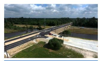
The addition of a bike path provides accessibility and safety for pedestrians while the drainage improvements reduce the risk of road flooding and water hazards for motorists.
