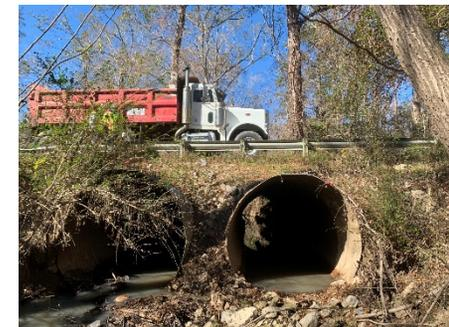
Live load tests were performed to aid in evaluating the structures in their current condition. The overall goal of these tests was to better understand the structure’s behavior and in turn provide field-verified load ratings for each structure. To achieve this goal, the collected structural responses were used to generate a field-verified finite-element model (FEM) of the structure.
