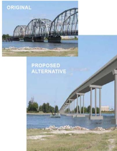
Arcadis was contracted by LADOTD to complete preliminary **design layouts to replace the existing US 90 swing- span bridge** over Chef Menteur Pass in Orleans Parish as part of an **environmental assessment**. Both movable- and fixed-span designs were considered along with three preliminary alignments. **LADOTD Design Guidelines and EDSMs** along with the **LADOTD Road Design and Bridge Design Manuals** were utilized.
